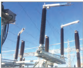
HV CIRCUIT BREAKERS - HV DISCONNECTORS (up to 420kV)
