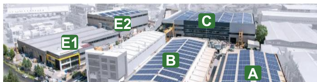
(A) TURKAK-accredited HV test lab, largest of its kind in Turkey, meeting international technical standards
