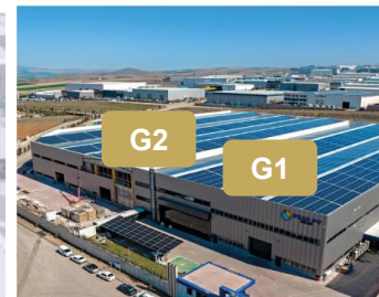
(G) Solar panel production & mounting systems
